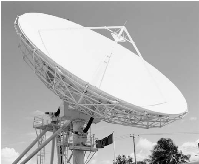
Figure 2.15 Satellite ground station (Courtesy Cable and Wireless)
