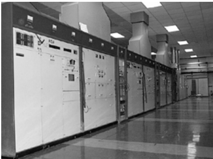
Figure 2.4 High power Medium Wave transmitters at Brookmans Park transmitting station (Courtesy Crown Castle International)
