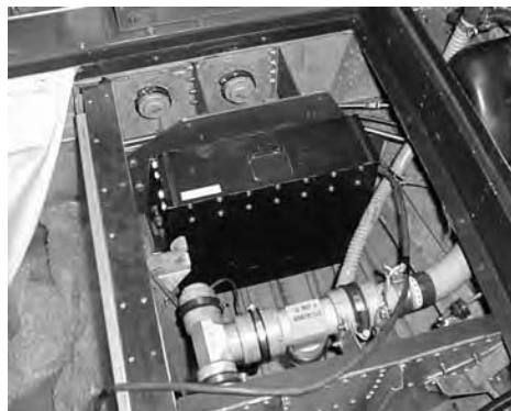
Figure 12.24. Implementation of a generator on a prototype. Photo: Eurocopter
