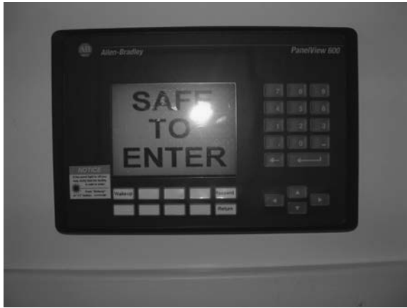
FIGURE 14.41 Interlock system.
