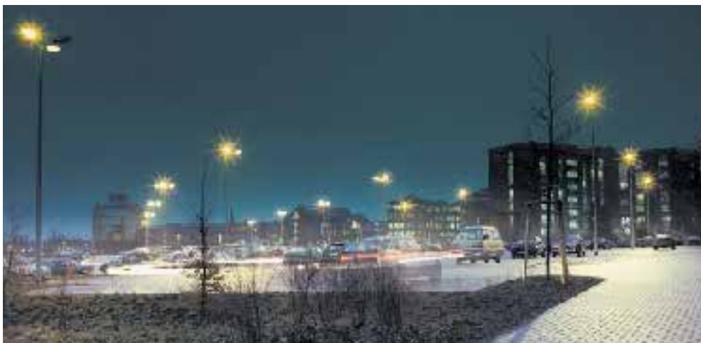
The arrangement of parking spaces dictates the arrangement of luminaires. Mounting heights up to 12 metres are suitable for lighting a large outdoor car park like this. 77
