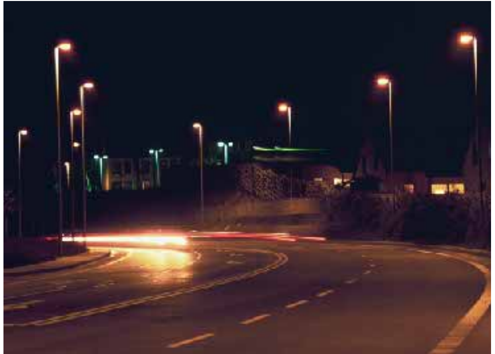
Where luminaires are single-lamped, the only acceptable way to power down to a lower night-time lighting level is to reduce the connected load of each light source. 101
