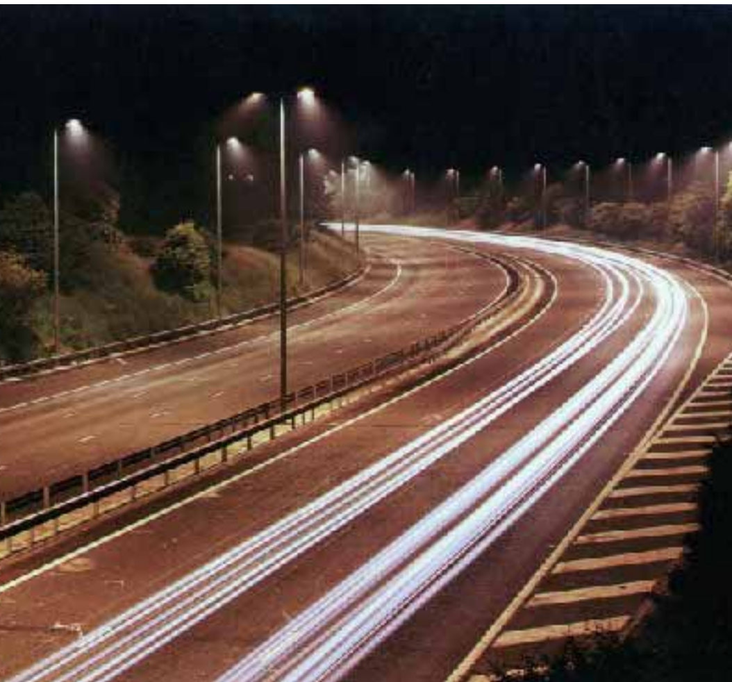
On the bend, luminaires are not positioned on the central reservation. Closer luminaire spacing in the middle of the bend makes for a better "guide-rail" effect. 38
