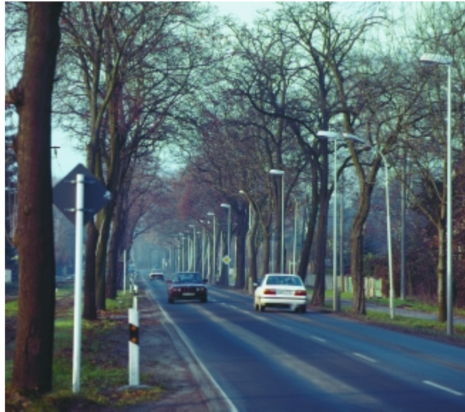
A link road between two villages with lighting designed to DIN 5044 specifications. 39
