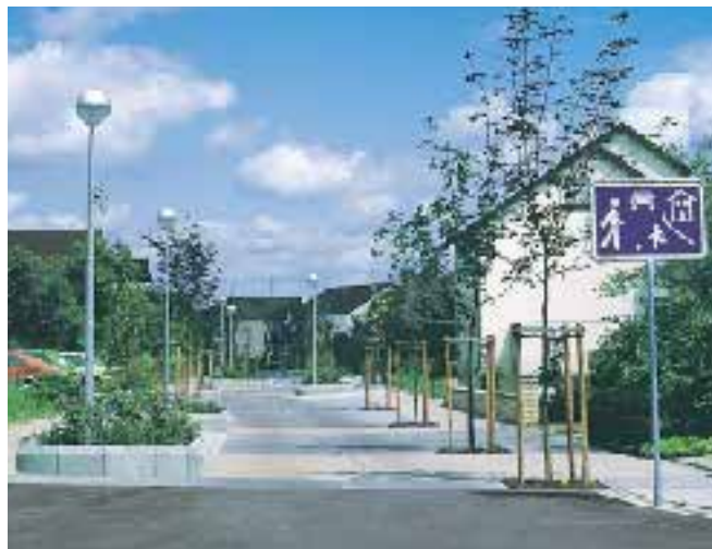
Quality lighting even where nothing moves faster than walking pace: globe luminaires in a traffic-calmed street.
