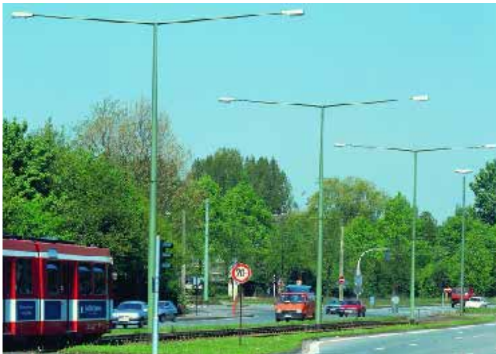
Hazard zones on a road are highlighted by supplementary lighting – here provided by the luminaire in the background on the right.
