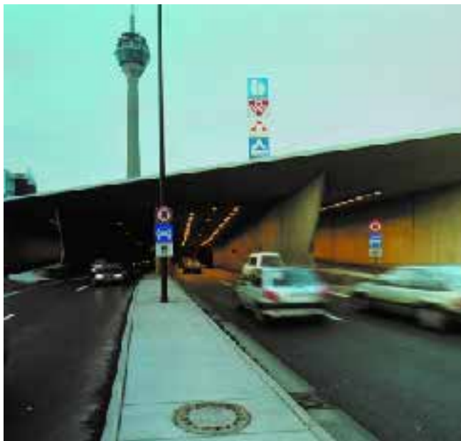
From outside, a tunnel entrance looks like a black hole. A high level of lighting dispels that impression and makes it easier for our eyes to adapt. 78
