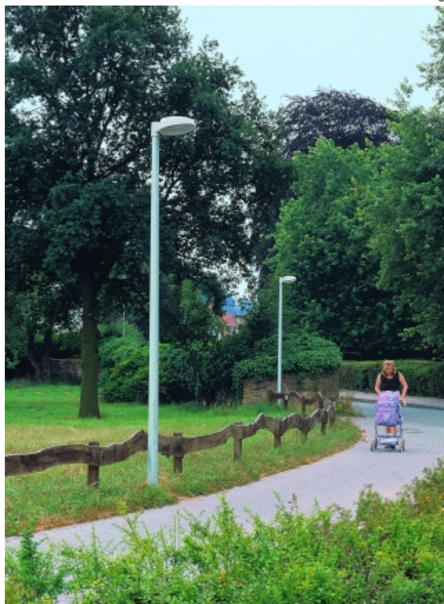
The lower the mounting height, the closer the spacing required between luminaires.
