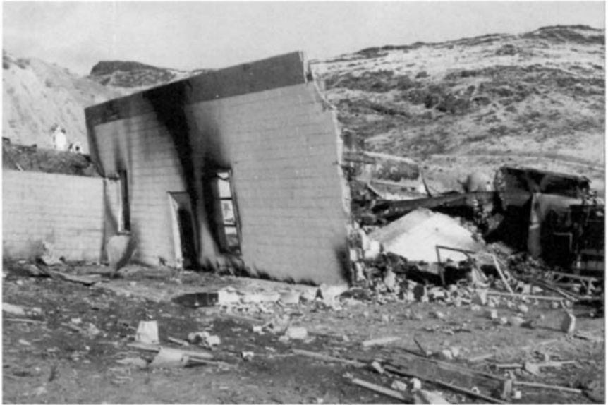
Figure 6–9 Remains of Booster Room 1 of the Sierra Chemical Company Kean Canyon plant east of Reno near Mustang, Nevada, USA, after explosives mix explosion in 1998. From CSB (1998).
