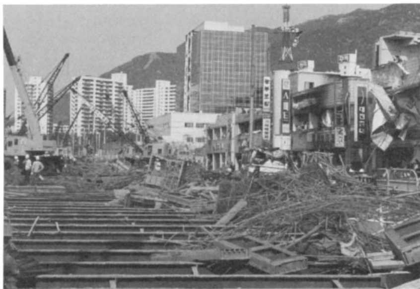
Figure 2–58 Site of the LPG explosion disaster in Taegu, South Korea, April 28, 1995, which killed 100 people, and injured 117. Ten buildings were completely demolished and 48 others partly damaged, while 80 vehicles were destroyed or damaged. From Fire Investigation Report (1995).
