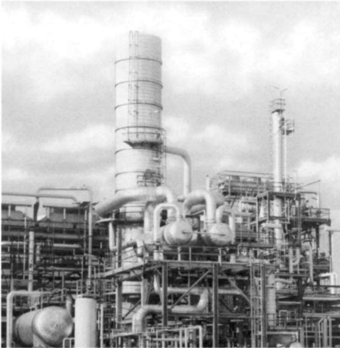
Figure 2-69 Highly congested process plant in which very high explosion pressures can be generated in case of a gas explosion.
