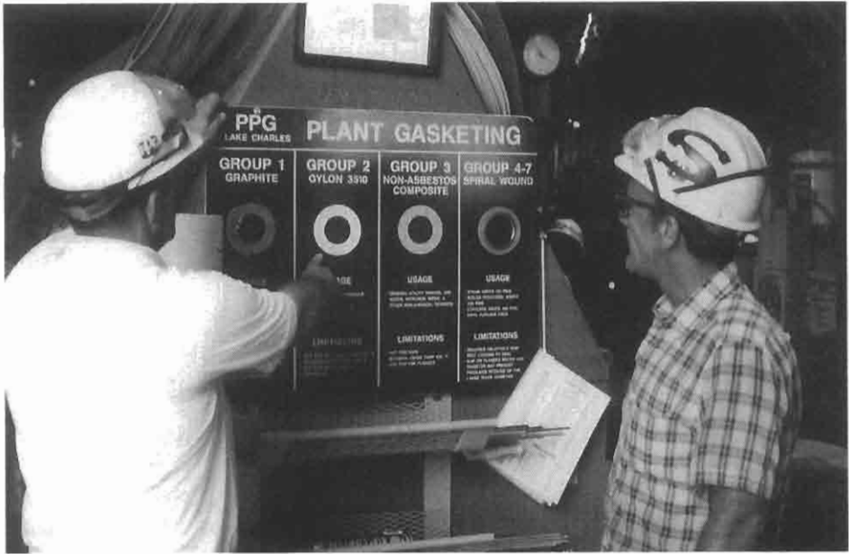
FIGURE 6-9 Choosing the proper piping gaskets with help from easy-to-understand gasket board.
