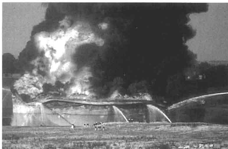
FIGURE 7-2 A fire in a giant floating roof crude oil tank. Courtesy of the Institution of Chemical Engineers. This photo is from Hazards Workshop Module 006, "Preventing Emergencies in the Process Industries."
