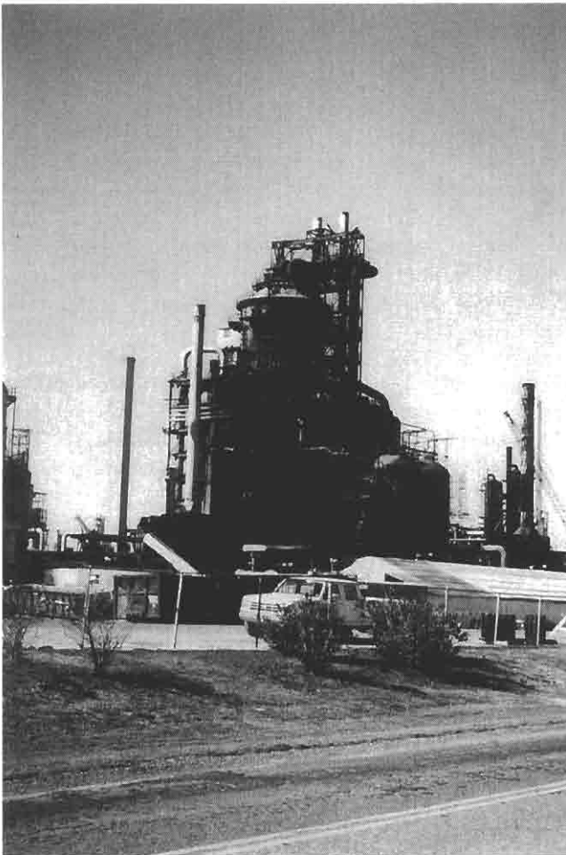
FIGURE 3-12 After the explosion, a charred multi-storied catalytic cracking unit.
