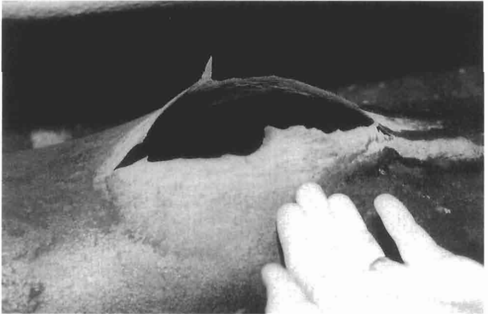
FIGURE 6-3 Close up of the tube failure.
