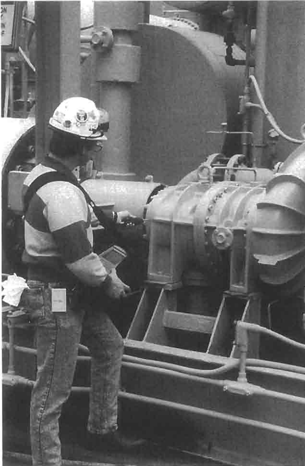
FIGURE 9-3 A vibration technician taking readings on a refrigeration compressor.
