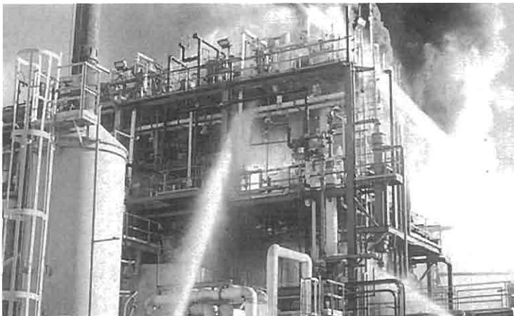
FIGURE 7-7 Fire intensely burning in the reactor area in the third level of structure, while hose streams supplement the fixed water spray. Courtesy of G. O. Heintzen.
