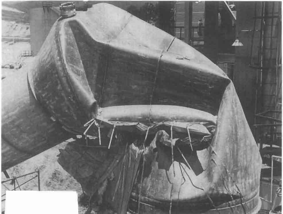
FIGURE 3-7 A close-up of a collapsed stripper column. Courtesy of Guido DeJesus.
