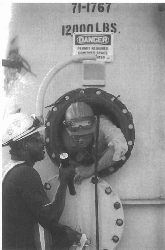
FIGURE 9-10 A pressure vessel inspector enters the confined space after the vessel is blinded, tested, and cleared, but still relies on a manway watch.
