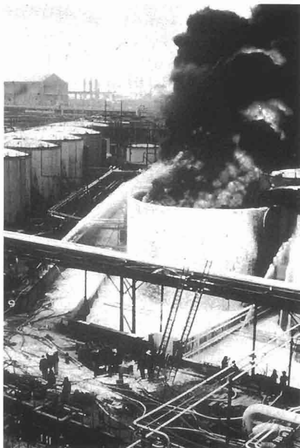
FIGURE 7-3 After the top opened, a fire burned but the liquid was still contained. Courtesy of the Institution of Chemical Engineers. This photo is from Hazards Workshop Module 003, "Fires and Explosions."
