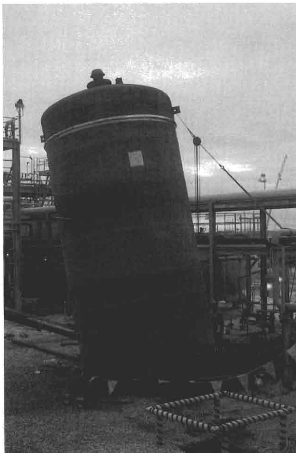
FIGURE 5-11 A large acid tank fails due to blocked vent and a blocked overflow line.
