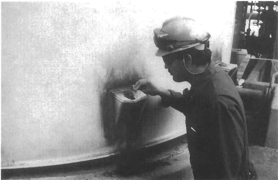
FIGURE 3-4 Tank bottom is bulged and anchor nuts are pulled through the anchor chairs.
