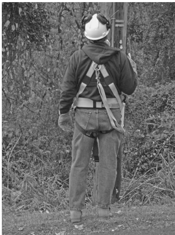
FIGURE 25.12 Worker wearing a personal fall arrest system.
