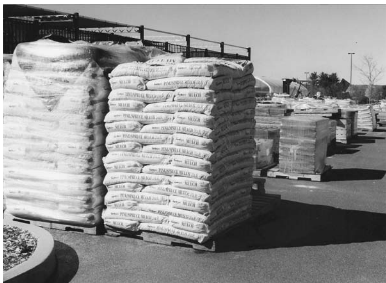
FIGURE 25.22 Example of adequately stacked materials.
